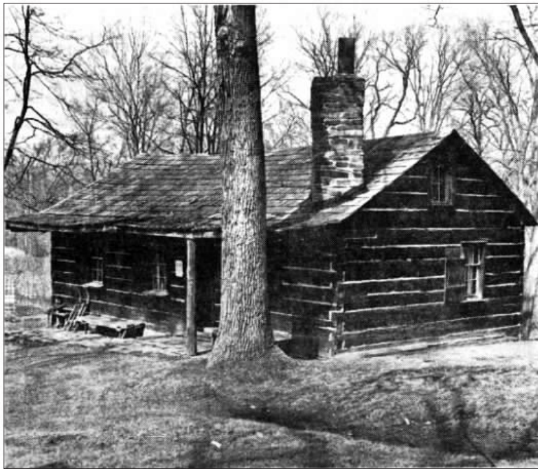
CABIN IN THE SUN —This cabin of hand-hewn logs stands along Pumpelly Creek in Tioga County and is owned by Spencer A. Pumpelly, 44 Front Street, Owego. Mr. Pumpelly discovered the cabin, built about 1815 by a settler named Bill White, near the settlement of Waits close to the Pennsylvania border. Mr. Pumpelly took the cabin apart, log-by-log, in 1939, moved it to its present location and reassembled it.
